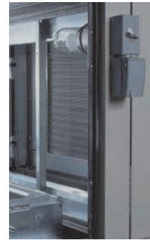
Lights and receptacles
