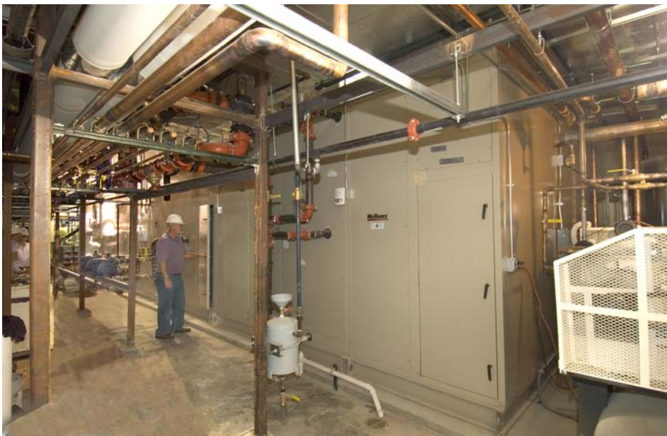
One extended-size Vision air handler serves the building's entire east wing, significantly reducing installed costs and operating costs.
