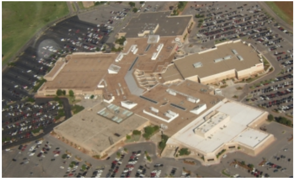
McQuay rooftop units supply heating, cooling and ventilation to Quail Springs Mall, Oklahoma City.
