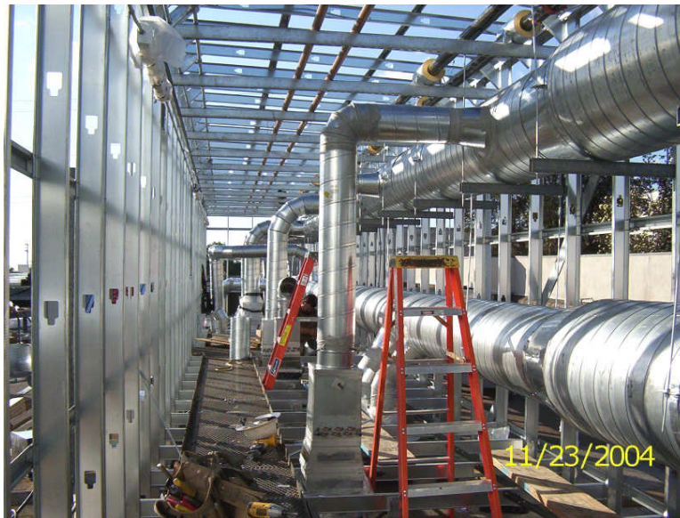
Figure 8: New penthouse for new VAV air-handlers
